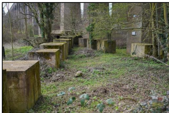
Chappel Viaduct. W. Shepherd
